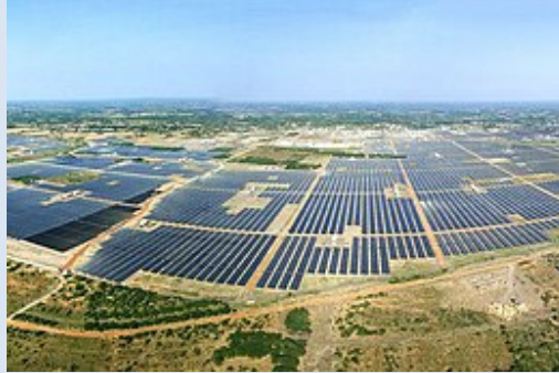
Aerial view of Kamuthi Solar Power Project
